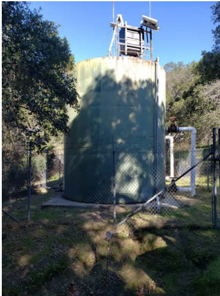
Photo 1 – Existing Ballantree Storage Tanks
