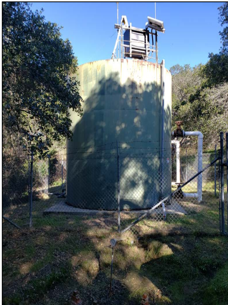
Figure 2-8 Ballantree Storage Tanks
