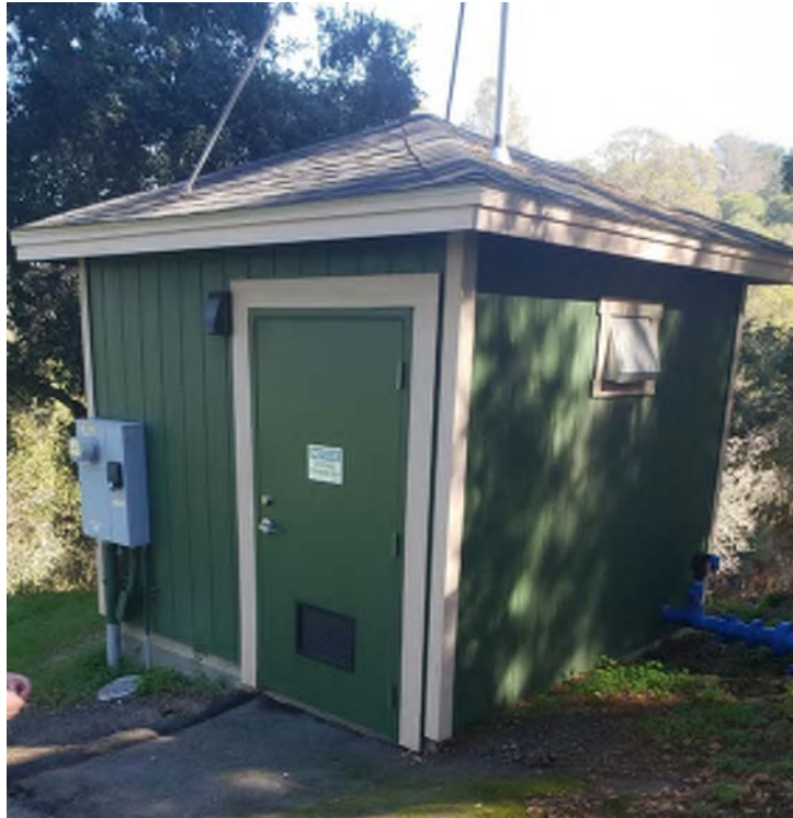
Photo 2 – Oakridge Pump Station
